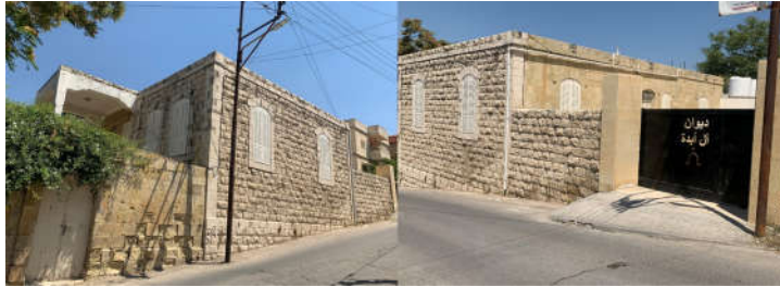
Figure 16: Image of Abida House, shows the two entrances of the house, two types of stone were used in construction too. Source: captured and appropriated by the researches 2020
