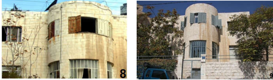
Figure 8, 9: before and after image of the main elevation of the building.
