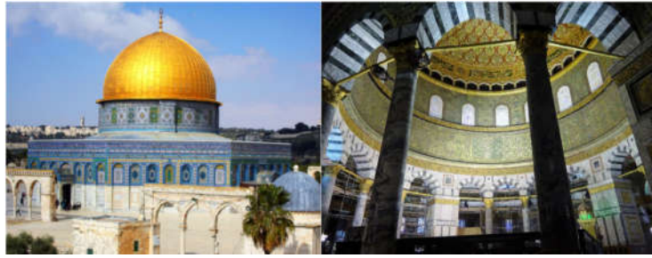
Figure 12: The Dome of the Rock, Exterior & Interior (www.domeoftherock.com)
