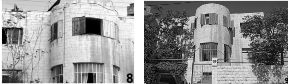
Figure 8, 9: before and after image of the main elevation of the building.
